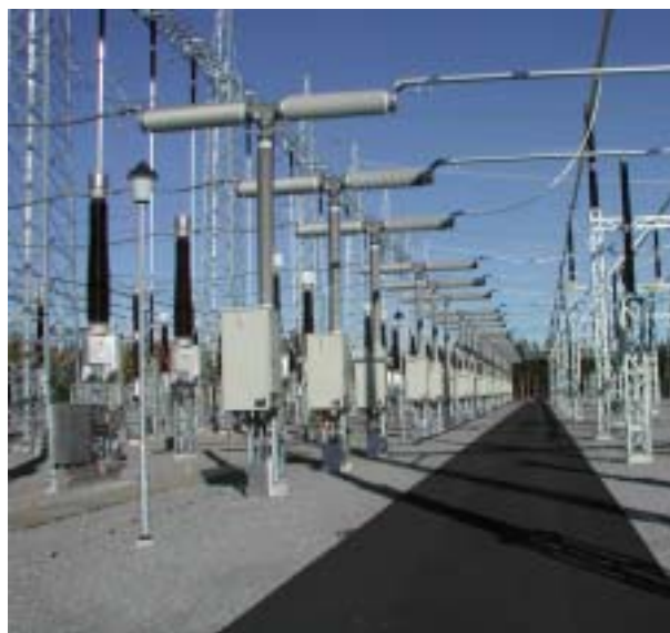
The new Swedish "Combined breaker" contains both disconnect and breaker. Photo: Pentti Lehto
