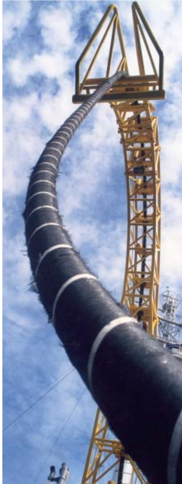
Cable installation. Photo: Trond Isaksen
