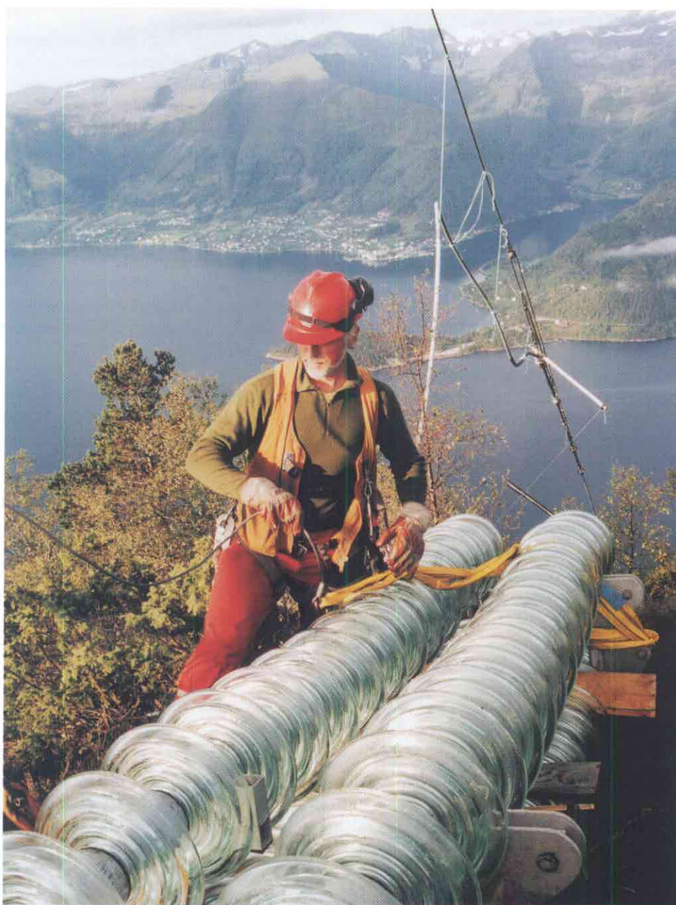
Statnett carries out its biggest distribution project so far by constructing lines to span 30 Norwegian fjords. Lines were fixed and insulated on the power line across the Fjærland Fjord in autumn 1997. Photo: Einar Kr. Holtet.
