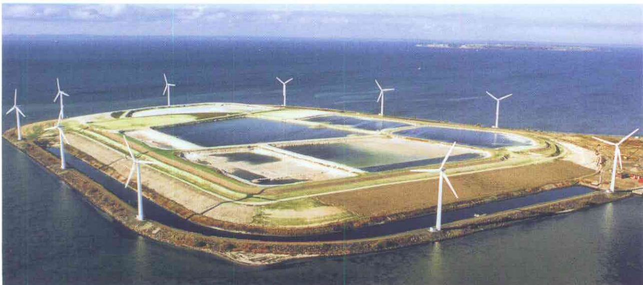
In 1996, Sydkraft commissioned 12 wind power plants on Gipsön island, off Landskrona. Each plant has a power rating of 600 kW. Photo: Perry Nordeng
