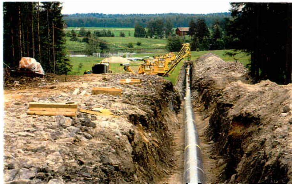
**Figure 7 Laying a natural gas pipeline in forested ground**
